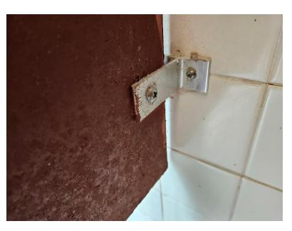
The second floor ladies' room has taken a beating since 1985. The stalls and hardware are rusted. The Township had to build the legs for the sink as the old components broke due to heavy use and children being set on the sink counter. The sink pipes are exposed and many floor tiles are broken. The ventilation is very poor. As noted in the photos, neither stalls are ADA compliant.
