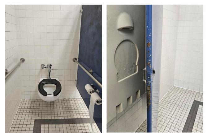
The second floor mens' room has fared slightly better over 38 years. However, the stall is only ambulatory, not ADA compliant. The stall wall, door and fixtures are rusted. There is no new construction for the second floor restrooms.
